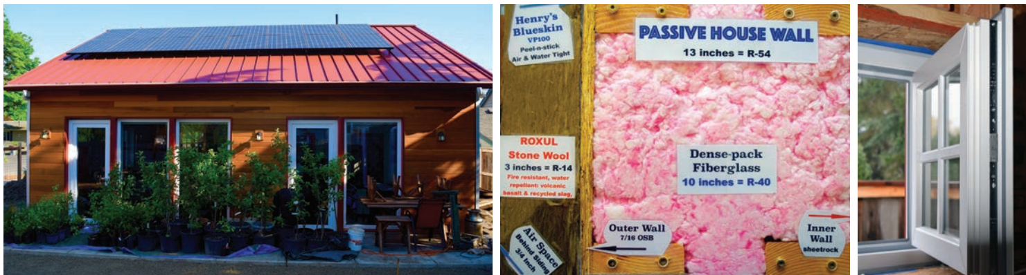
Efficient to the extreme ✧ The Pitneys' "forever house" features rooftop solar panels, 13-inch exterior walls and triple-pane windows more than 3 inches thick
